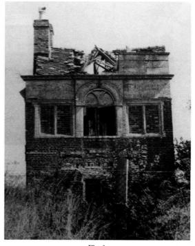
Fig. 1 The Warren House at its lowest ebb, in 1985. A temptation to vandals, the roof has caved it and its triangular pediment has collapsed. *Photograph*, TAMS, 29 (1985), 166
